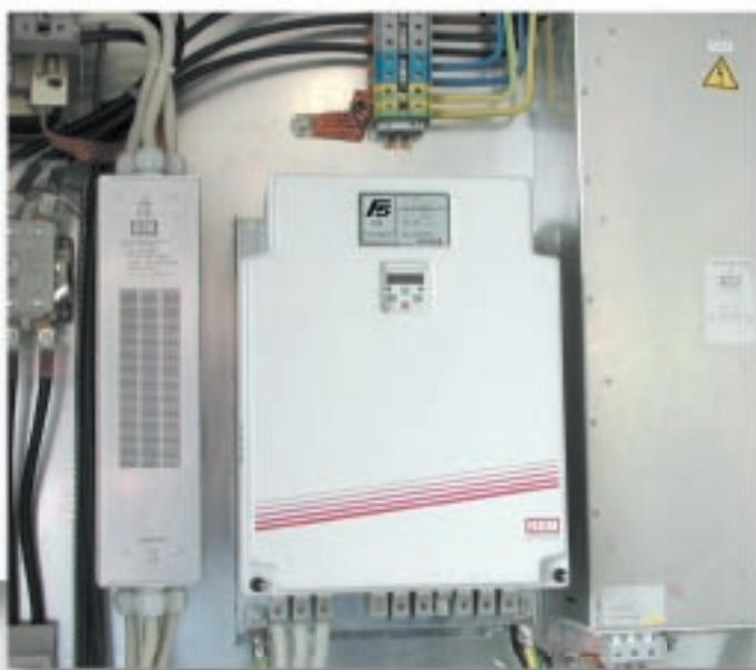
For inverters with a rated power of 90 kW and above KEB offers a **book-style side-mount filter**
